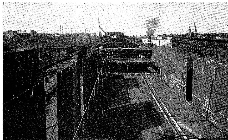
First of the three new Pittsburgh ships to be completed will be “Hull 867”, shown here after 42 weeks of work at the Lorain yard of American Ship Building Co. There is lively conjecture in shipping circles as to whether this ship or Cleveland Cliffs’ E. B. GREENE, going up at Toledo, will be first to join the Great Lakes fleet.
