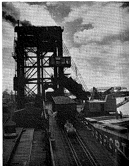
A full carload of 60 tons at a time is dumped into vessels by coal loading facilities of the Great Lakes such as this one pouring cargo into the McFarland at Toledo.
